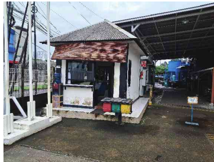
Tampak Depan Bangunan Pos Jaga Front of the Guardhouse Building
