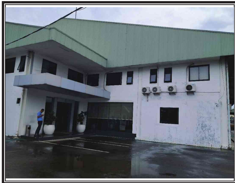
TAMPAK DEPAN BANGUNAN KANTOR FRONT VIEW OF OFFICE BUILDING
