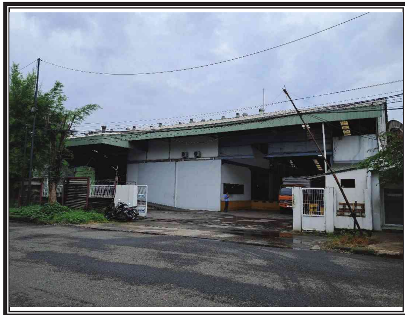
TAMPAK DEPAN BANGUNAN PABRIK FRONT OF THE FACTORY BUILDING
