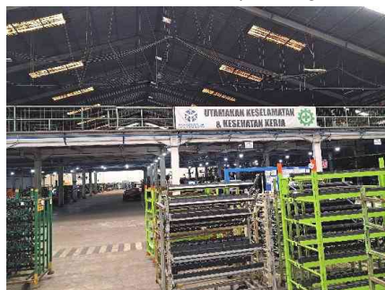
Tampak Bangunan Mezzanine Front of the Mezzanine Building
