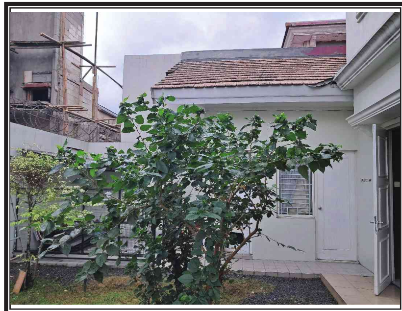
TAMPAK HALAMAN BELAKANG CONDITION OF THE BACKYARD AREA
