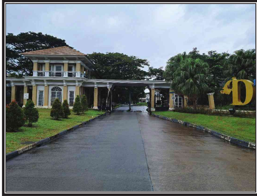
SITUASI GERBANG MASUK KOMPLEK CLUSTER ENTRANCE GATE OF THE RESIDENTIAL CLUSTER
