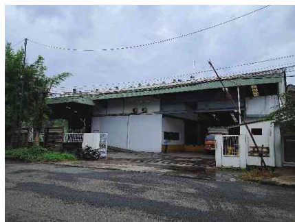
Tampak Depan Bangunan Pabrik Front of the Factory Building
